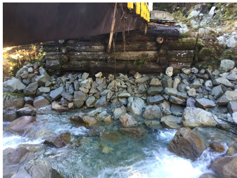
Right Bank Abutment when facing downstream
