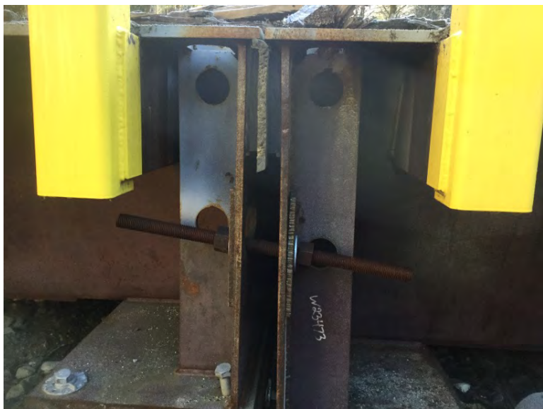
Pier superstructure connection
