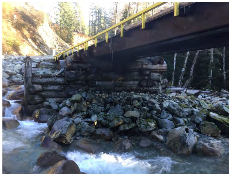
Right face of pier
