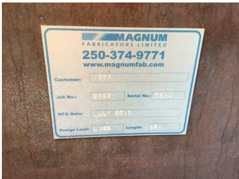
Right span structure ID
