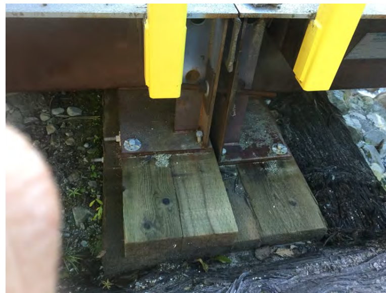
Upstream pier bearings
