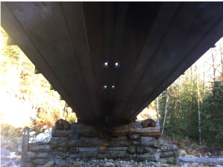
Right span superstructure
